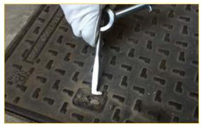
$\begin{tabular}{ll} \textbf{Configuration 2:} L - shaped end for scraping in the inside of the slot and release the rotation for opening the lid. \\ \end{tabular}$
